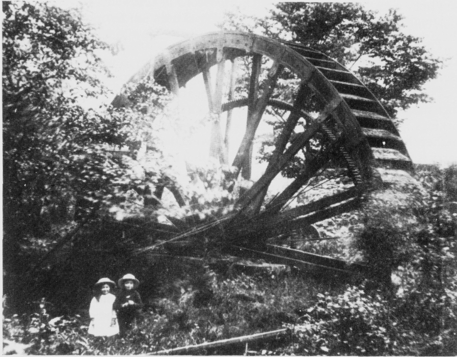
Fig. 3 Waterwheel, Park Village Limeworks, about 1900-1910. Note the two gear rings — the smaller probably for haulage, the larger for blowing.
