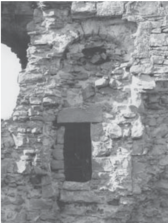
Fig. 3 Torthorwald Castle. Detail of window inserted in original entrance doorway of first floor.
