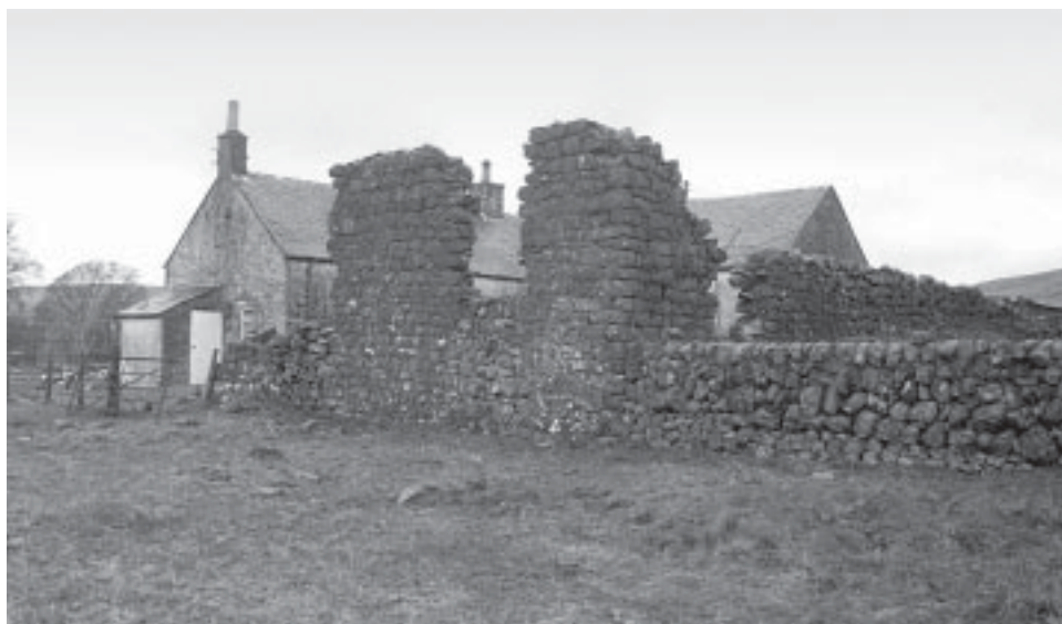
Fig. 2 Lagwyne Castle: General view, from the south, of surviving walls.
