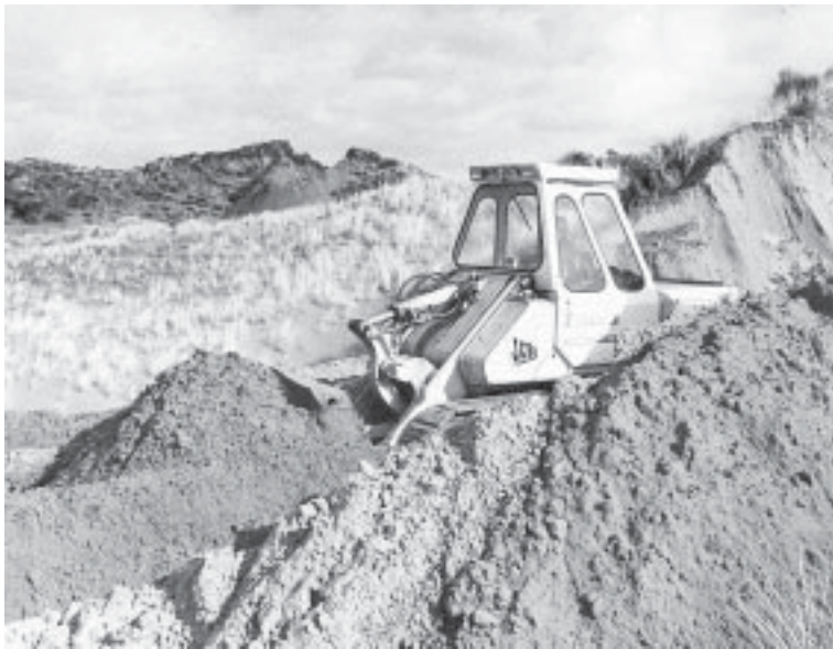
Figure 6 JCB 110 clearing overburden to expose buried soil at Site H.
