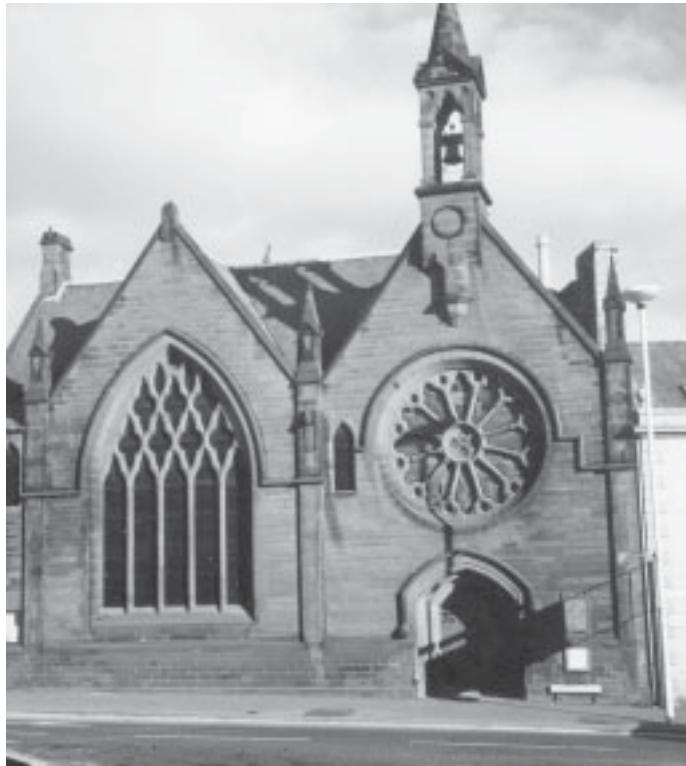
Fig. 5 View of Townhead South Free Church, Nith Place, Dumfries: built 1862-5, demolished 1995. (Photo, A.C. Wolffe)
