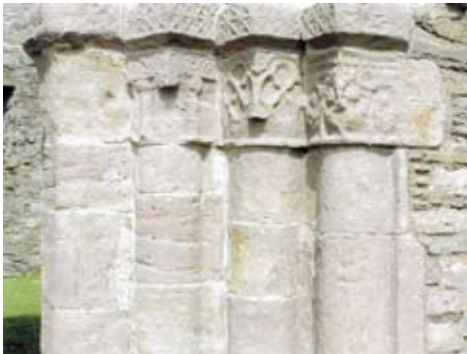
Figure 3 Whithorn Priory – 12th century doorway detail, using Wall Hill, Netherlaw sandstone
