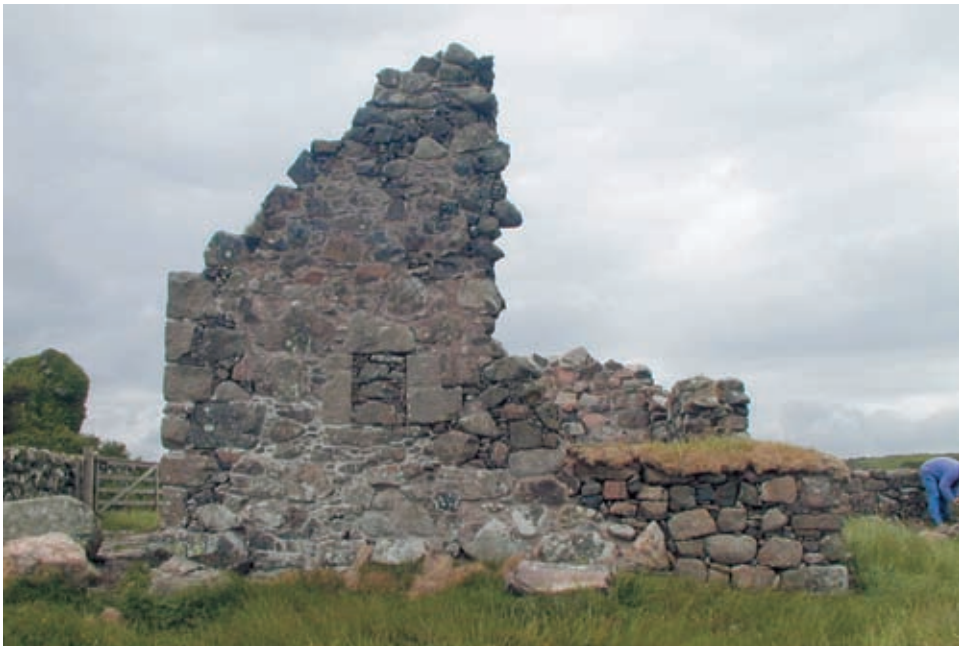
Figure 11 Building A from south after consolidation
