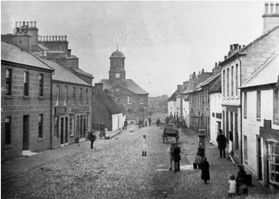
Figure 1. An early photograph of Sanquhar High Street, facing north-west. The photograph is believed to date from the 1860s and certainly predates construction of the Town Hall, completed in 1882, which stands beyond and to the right of the 1735–7 Tolbooth. On the extreme right of the picture is the bow-windowed Post Office, and the frontages on that side of the street are those described on the previous page. On the opposite side, the tall building set back from the road is shown on the Ordnance Survey 25-inch map of 1860 as a branch of the Western Bank of Scotland, acquired by the Royal Bank when the Western Bank collapsed in 1857. The thatched house beyond it is the first in a row of three, as shown on the 25-inch map; as late as 1837 such single-storey thatched houses were common in Sanquhar 11 . (Courtesy of Dumfries Museum)
