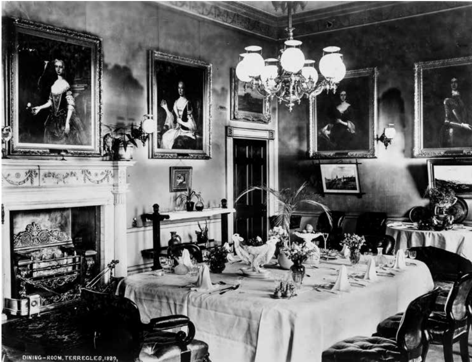
Figure 30. Interior Rooms 1889. Most of the photographs in the collection are external shots of properties. These scenes at Terregles House, in contrast, provide an insight into the furnishings and style of grand Victorian mansions. The Dining Room. (Album 2, number 45)
