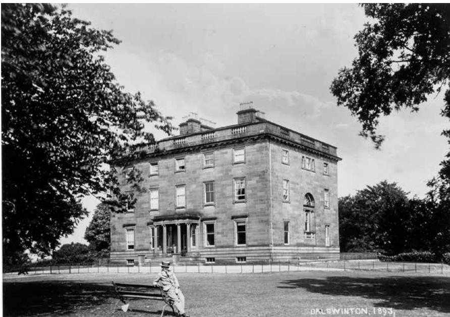
Figure 21. Dalswinton House 1893. ‘The central portico was replaced by a bow window to a design by Barbour and Bowie in 1919–20 and an extension was added on the north side where a new main doorway was installed.’ ( The Buildings of Scotland, Dumfries and Galloway by John Gifford, Pevsner Architectural Guides (London: Penguin Books) 1996). (Album 1, number 33)
