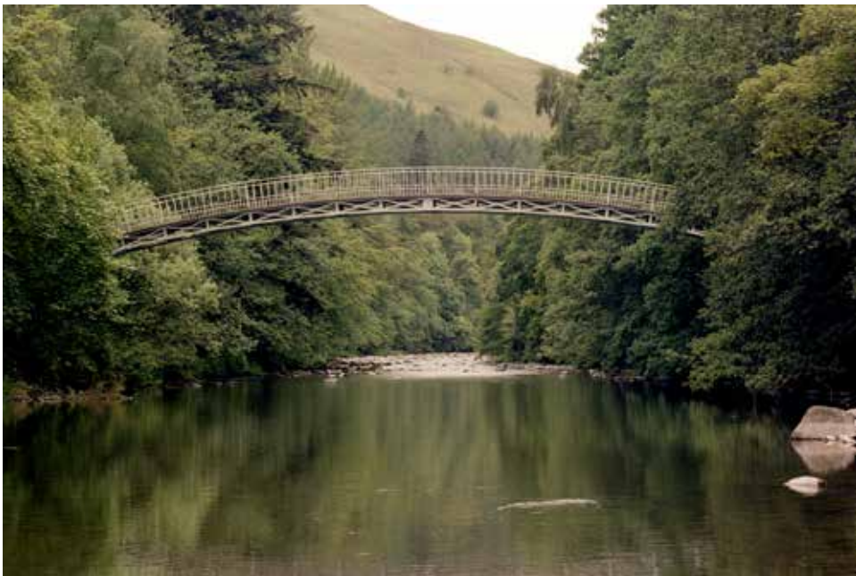
Figure 1. Duchess Bridge, Langholm in 1984, view from downstream showing the central portion. (Copyright RCAHMS SC 358518)
